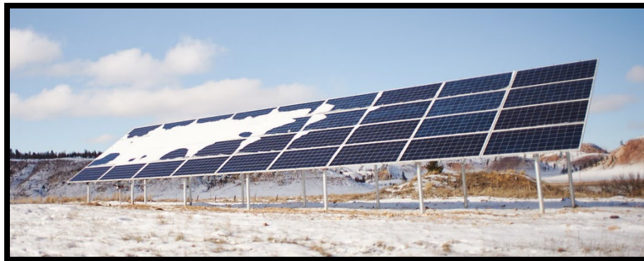
2 Figure 1. Muddy Hall PV array ( \alpha = 45^\circ , h = 48'' ) Feb 2, 2022 with significant snow cover. 1
